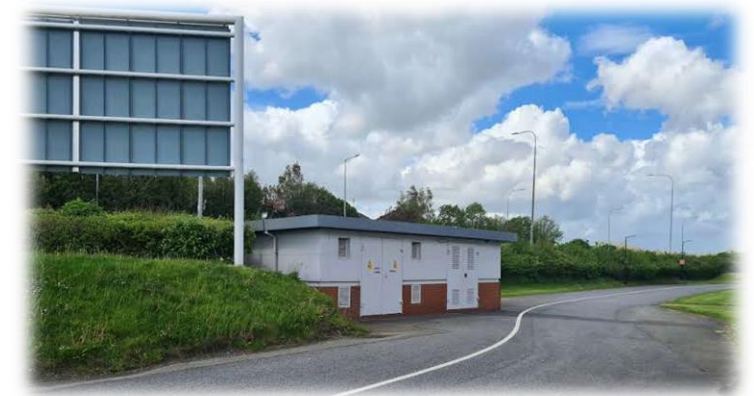
Substation to be moved at Airside Retail Park
