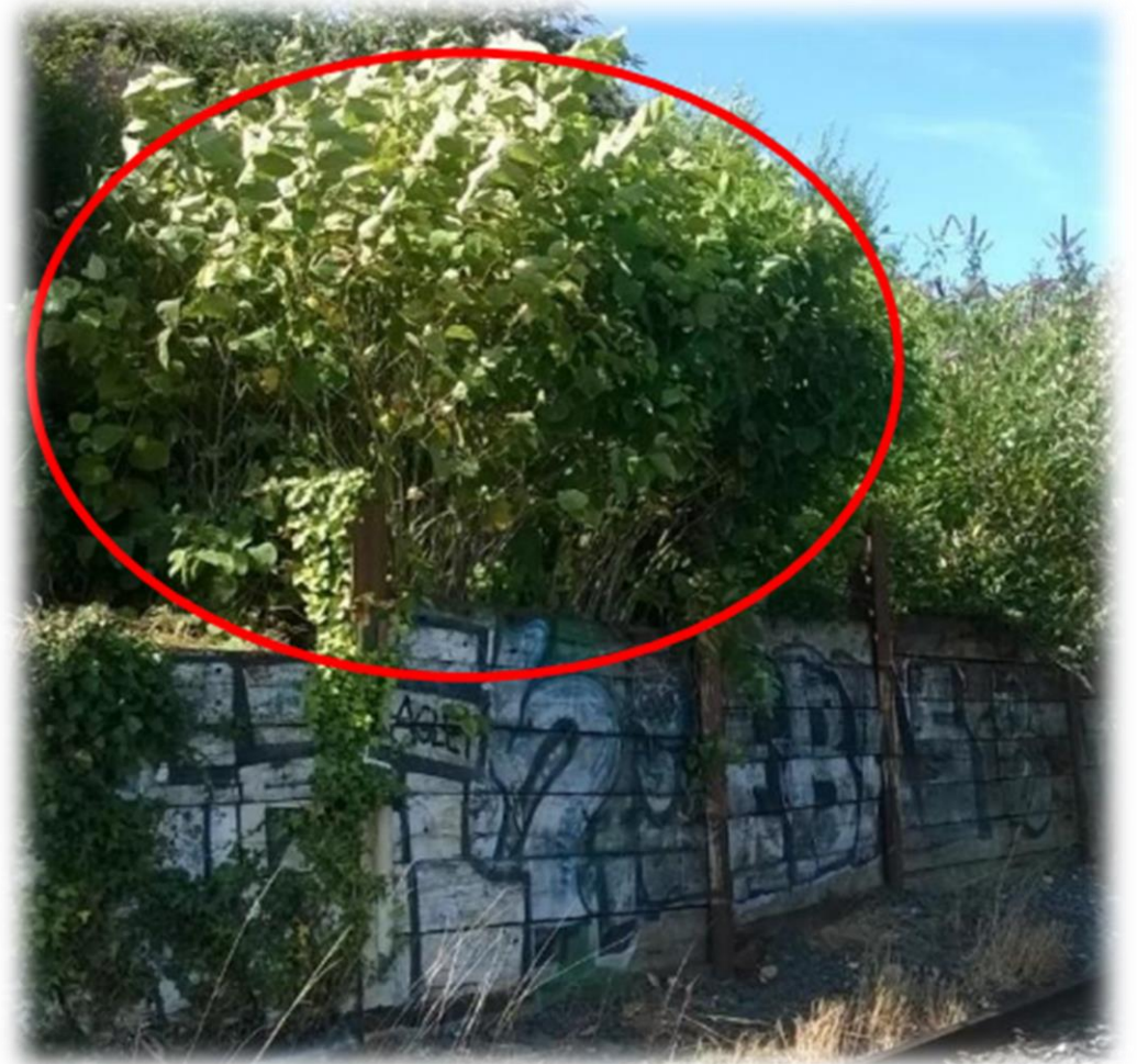
Typical Vegetation Clearance
